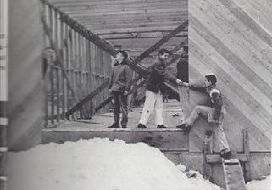
Inspection Crew--James Galbraith and Timothy Crowder view the "library" while Francis Freuchtl, Stephen Buckmaster and David Sheridan just arrive for the tour.
